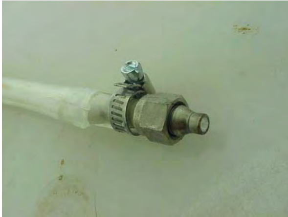
Injection End of Tubing
